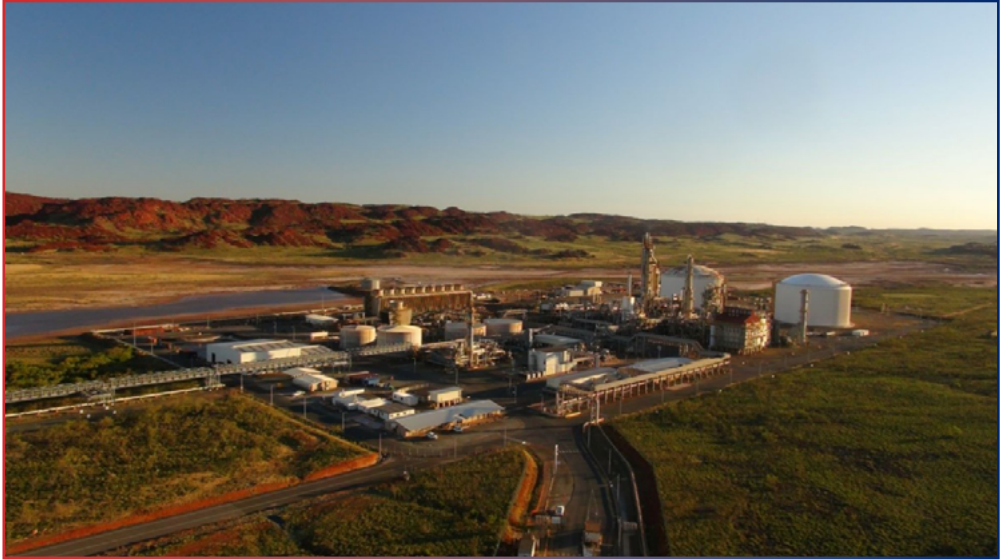
Picture 1: The Yara Pilbara ammonia plant in Western Australia. Source: Yara Australia Pty. Ltd.
